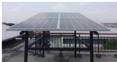
Fig. 1. Installation of 1 kW p of the SPP at ITENAS Bandung
